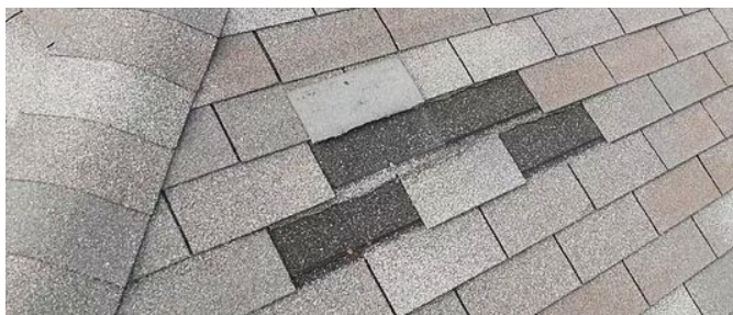
MISSING SHINGLES
