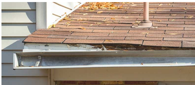
DAMAGED GUTTERS
